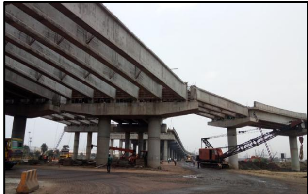
Fig. 15: A new Flyover under Construction
